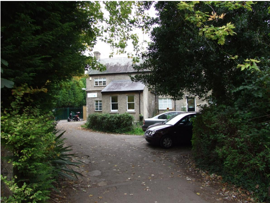
The former hall, now accommodating an International School
